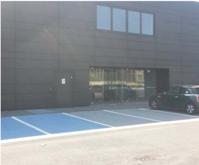
Building "I" outer front access
